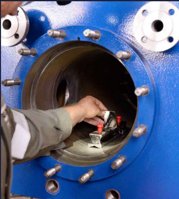
Overhaul of stage cylinders in Lingen & assembly on site
